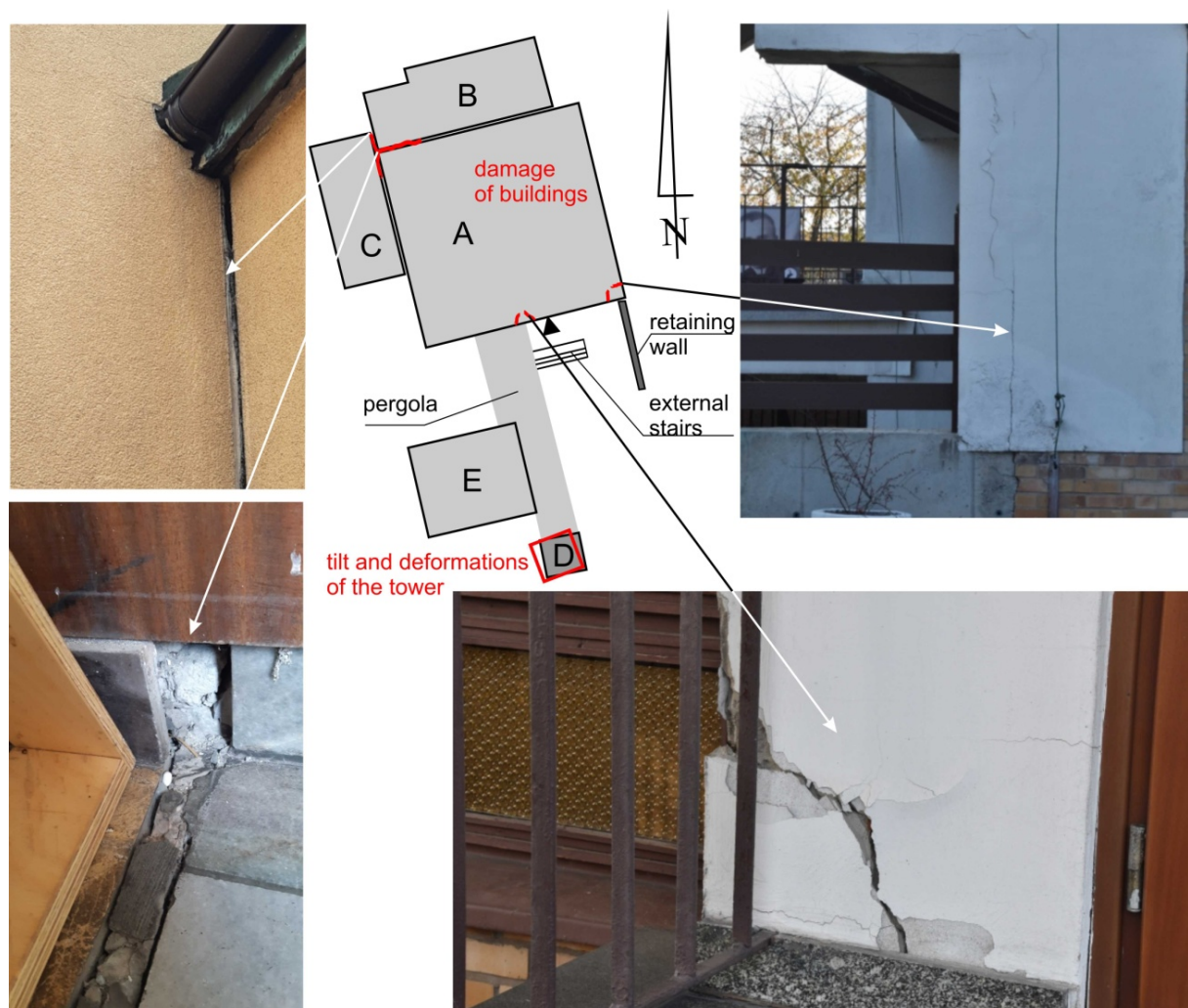
Figure 8. Damage and deformation observed in buildings
