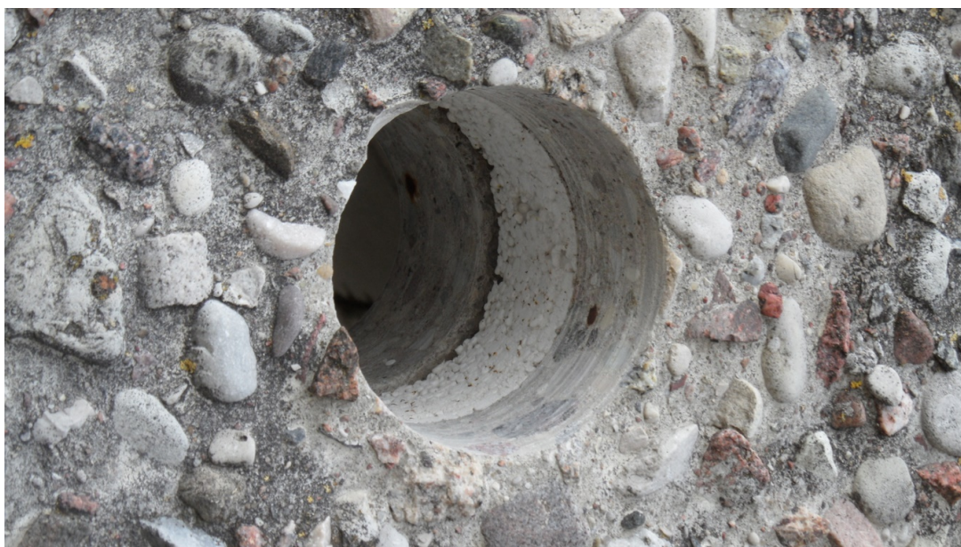
Figure 5. View of the hole made "through" using a drilling rig. [ref. own]
